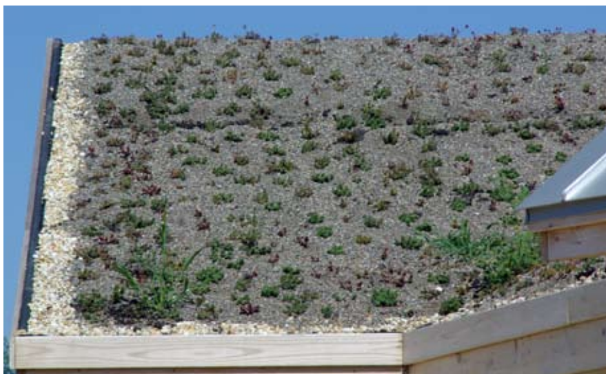
Black Ankle Winery's tasting room supports a living roof. Plants on the roof will cool the rooftop and absorb water resulting in less run off.
