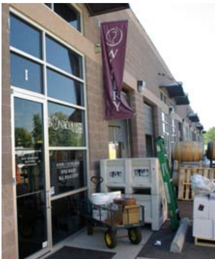
Bonacquisti Winery is built in a business park in Denver, Colorado.
